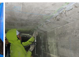
ひび割れ補修
